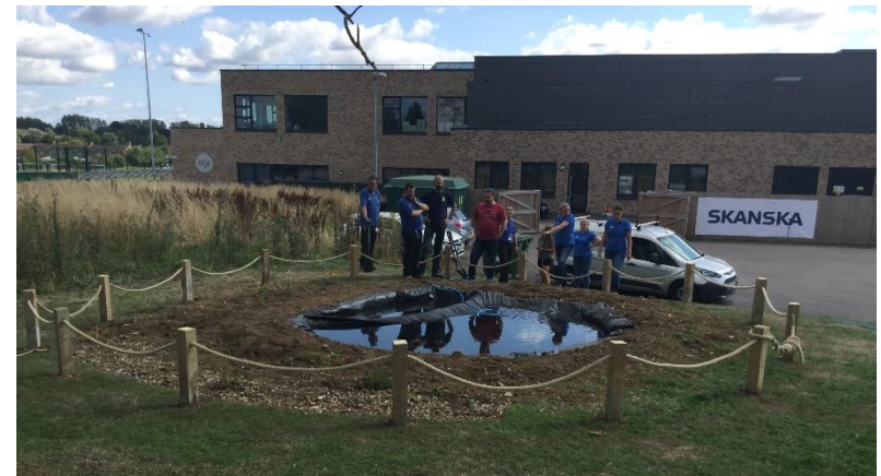
Following the installation of the new pond lining and fencing
