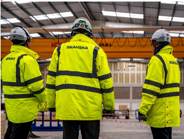
Facilities taking shape at VSSP.
